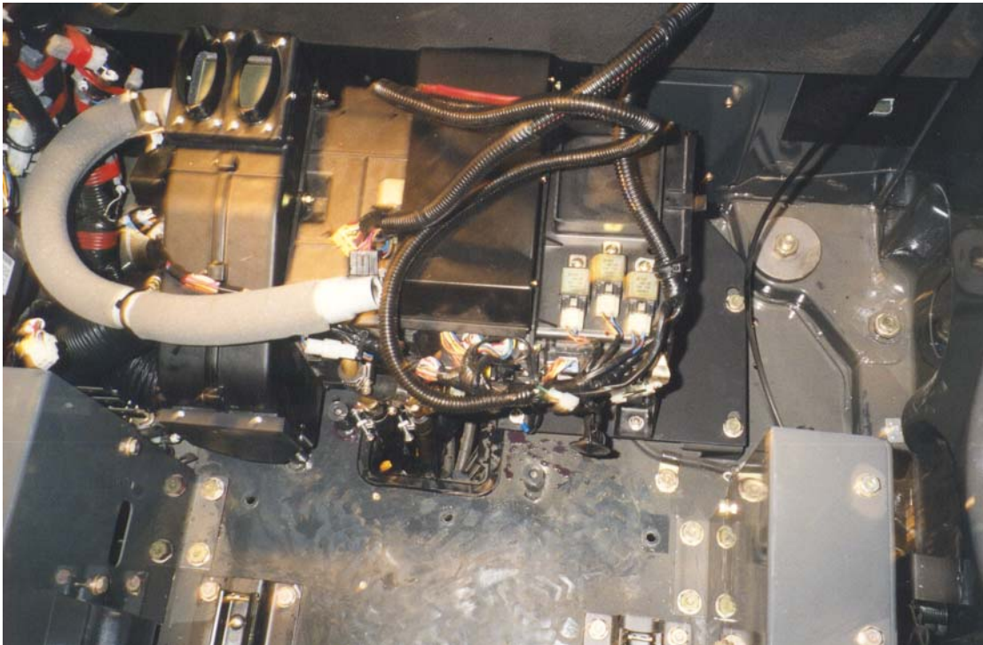
Evaporator assembly mounted in place.
